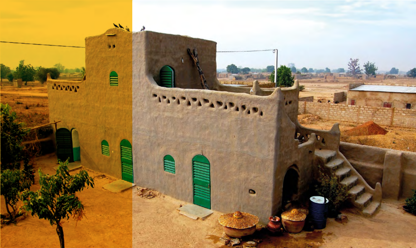
Examples of construction with a second storey.
